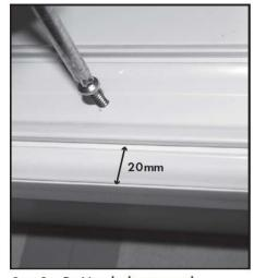
Step 2 - Position the bottom track ensuring it is placed 20mm in from the front of the wardrobe before securing. If a packer has been provided, this needs to be screwed/glued onto the hard surface under the bottom track first.
