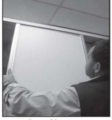
Step 3 - Slip top of door into rear channel then set bottom onto the rear floor track. Repeat for second door using front channel and track.
