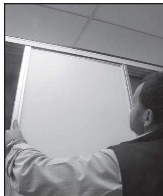
Step 3 - Slip top of door into rear channel then set bottom onto the rear floor track. Repeat for second door using front channel and track.
