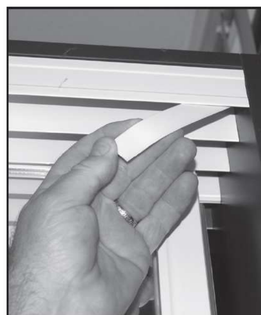
Step 6 - To control movement, peel adhesive & place the brake into each track where you want the wheels on top of the doors to remain stationary.
