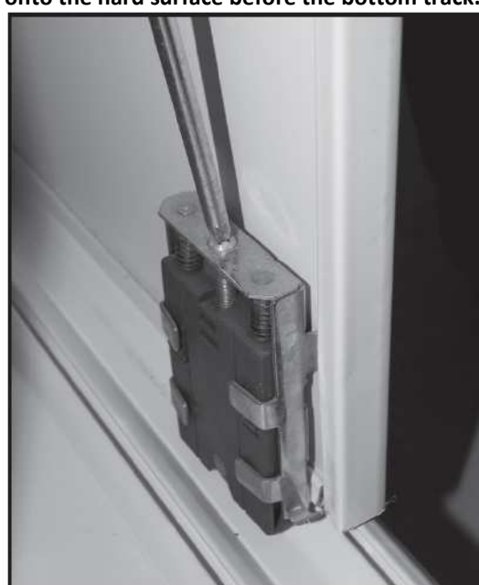
Step 5 - Adjust the ride height of each door with a Phillips screwdriver (clockwise to increase height).
