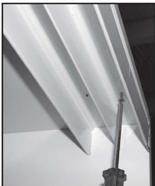
Step 1 - Position the top door track flush with the front of the wardrobe and secure using the screws provided.
