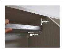
Measure the length between the installed rail brackets to get your rail length.
