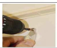
3. Mark on rail your measured length and cut the rail using a hacksaw. Once cut, slot rail into rail brackets.
