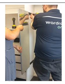
4. Once the top bracket is installed, simply line up the lower bracket in place and repeat steps 2 and 3 to fix the lower bracket in place.
