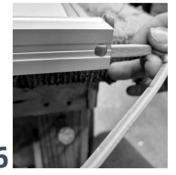
Starting at one end, slowly peel backing off and press strip position about 1 inch inside the door frame as shown. Gently pinch the buffer strip around the outside of the door frame, continue along pressing the buffer strip in place as you work towards the end. Repeat the same at the other end. Trim excess if required.
