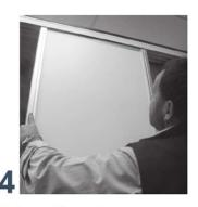
Lift the top of the door into the rear top channel, then set bottom wheels into the rear floor track. Repeat for the second door using the front channel and track
