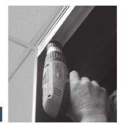
Align the top track flush with the front of your door jamb.
