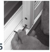
Use the 4mm allen key (provided) to adjust wheels to raise or lower the doors so they line up with side jambs. Clockwise adjusts the door height up, anticlockwise to adjust down.
