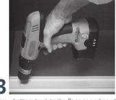
Screw bottom track to the floor or packer with the screws provided. Again, make sure it's 10mm in from the front of your door jamb.
