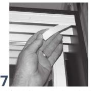
To help control movement, we have included a series of brake pads in the track pack. Peel the adhesive & place the brake into the tracks where you wish the doors to remain stationary.
