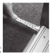
Position the bottom track ensuring it is placed 10mm in from the front of the wardrobe before securing. If a packer has been provided, this needs to be screwed/glued onto the hard surface under the bottom track first.
