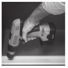
Screw bottom track to the floor with the screws provided. Again, make sure it's 10mm in from the front of your door jamb.
