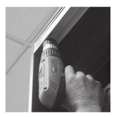
Fit the top track flush with the front of the wardrobe jamb and fix with the provided screws (5 screws for Double Top Track, 6 screws for Triple). Position screws 1-2 inches in from each end and space the rest evenly
