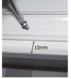
Position the bottom track ensuring it is placed 10mm in from the front of the wardrobe jamb before securing the remaining screws in the same positions as on the top track. If a packer has been provided, this needs to be screwed/glued onto the hard surface under the bottom track first.
