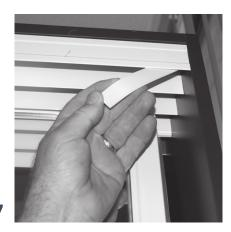
To help control movement, we have included a series of brake pads in the track pack. Peel the adhesive & place the brake into the tracks where you wish the doors to remain stationary.
