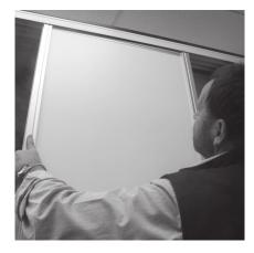
Slip the top of the door into the rear channel thenset bottom onto the rear floor track. Repeat for the second door using front channel and track.
