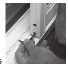
Use the 4mm allen key (provided) to adjust wheels to raise or lower the doors so they slide easily and line up with slide jambs. Clockwise adjusts the door height up, anticlockwise to adjust down.
